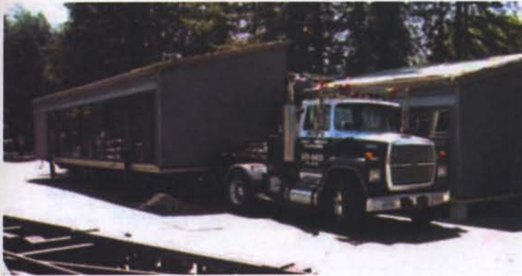
this page, top to bottom: Romero's LV, alternate plans; the LV flat-packed for shipment; mkd's Glidehouse modules in transit
