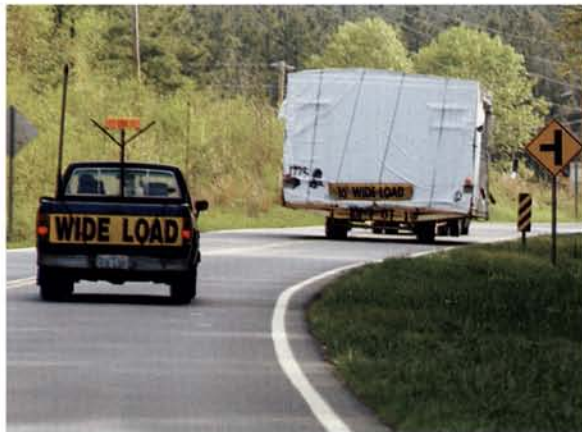
Left: Workers at Carolina Building Solutions prepare the modules for transport and then send them on their way. Below: The foundation in process.
