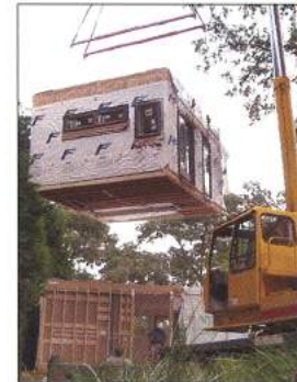
Cranes place Resolution: 4's second built modular house, in Annapolis, Md., onto its site (above). The firm's modular typologies (below) offer buyers a wide selection.
