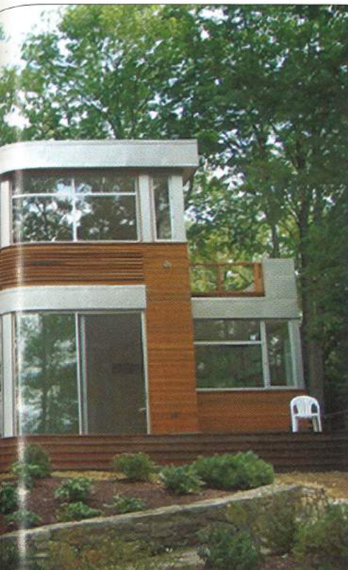
The floor plan and window placement at this conventionally constructed house in Kent, N.Y., help bring in lake and forest views.
