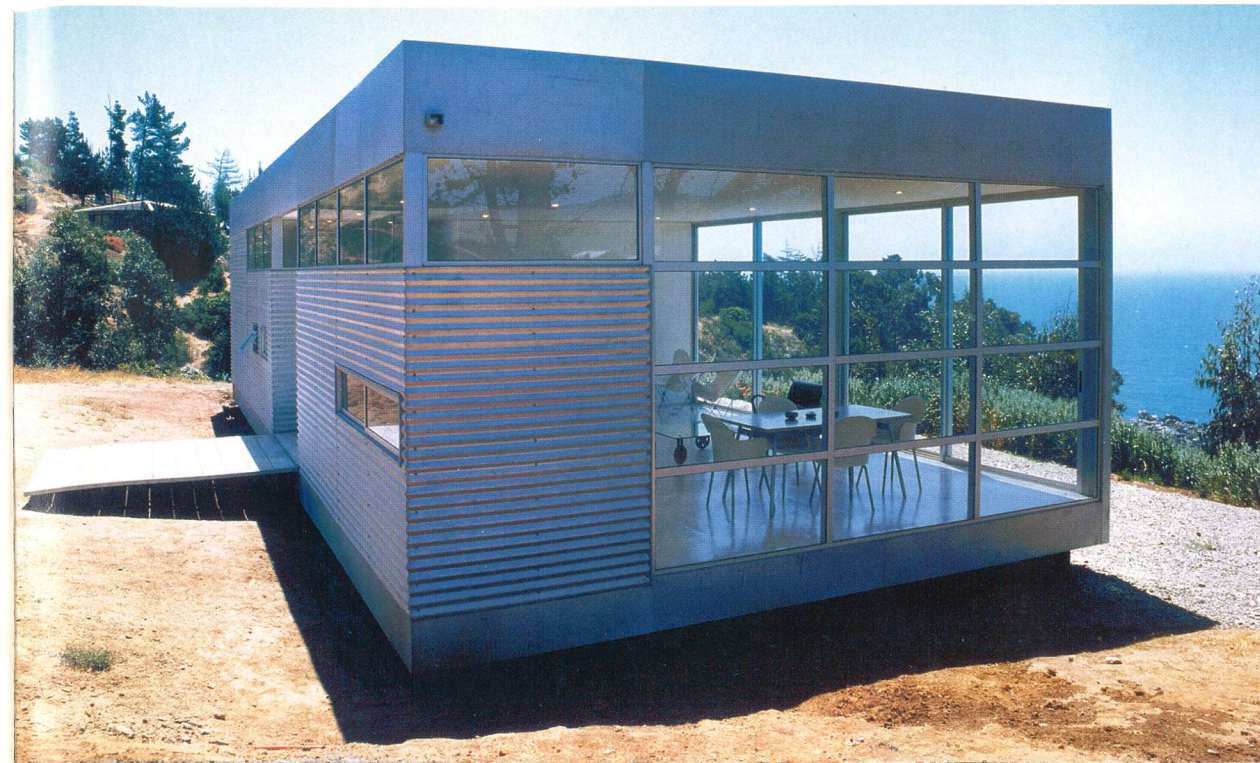
BUILDING BLOCKS: Romero's LV Home kit, left, is clad in corrugated aluminum; computer renderings of Siegal's Swellhouse, above, and the Dwell Home, by Resolution: 4 Architecture, below left; a 1941 version of Fuller's Dymaxion House, below; at bottom, workers in Pennsylvania assemble a prefab home in 1940
